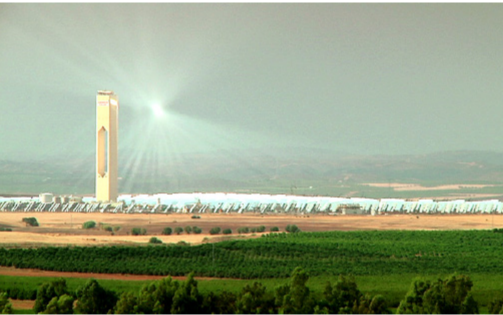
The Solucar Concentrating Solar Station, outside Sevilla, Spain, focuses the sun's heat on a receiver at the top of the tower.
