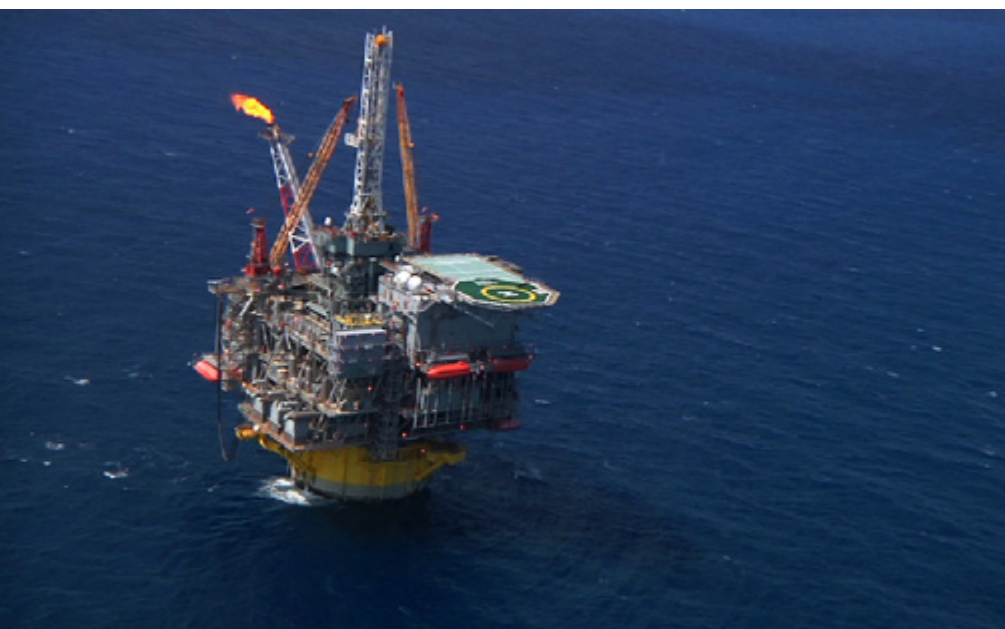
Perdido operates in the deepest water of any platform in the world, producing from 22 wells 8,000 feet below it.
